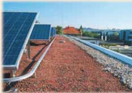
Non-penetration installation as the required load is provided by Zincolit® or system substrate or an alternative bulk material.
