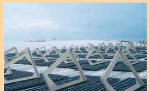
The Solar SGR 35/90 are placed on the ZinCo Solar Base® plates and adjusted.
