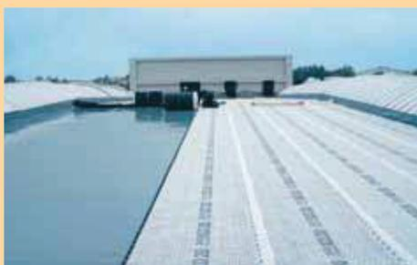
The roof membrane is covered with a Fixodrain® XD 20 high-grade drainage and protective layer.
