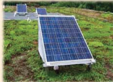
installed on “naked” bituminous panels being compared with one module installed on a green roof. In each case, attention was focused on the temperature at the underside
