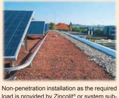
load is provided by Zincolit® or system substrate or an alternative bulk material.
