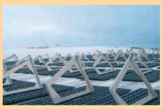
The Solar SGR 35/90 are placed on the ZinCo Solar Base<sup>®</sup> plates and adjusted.
