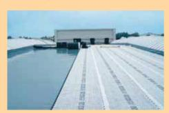
The roof membrane is covered with a Fixodrain® XD 20 high-grade drainage and protective layer.
